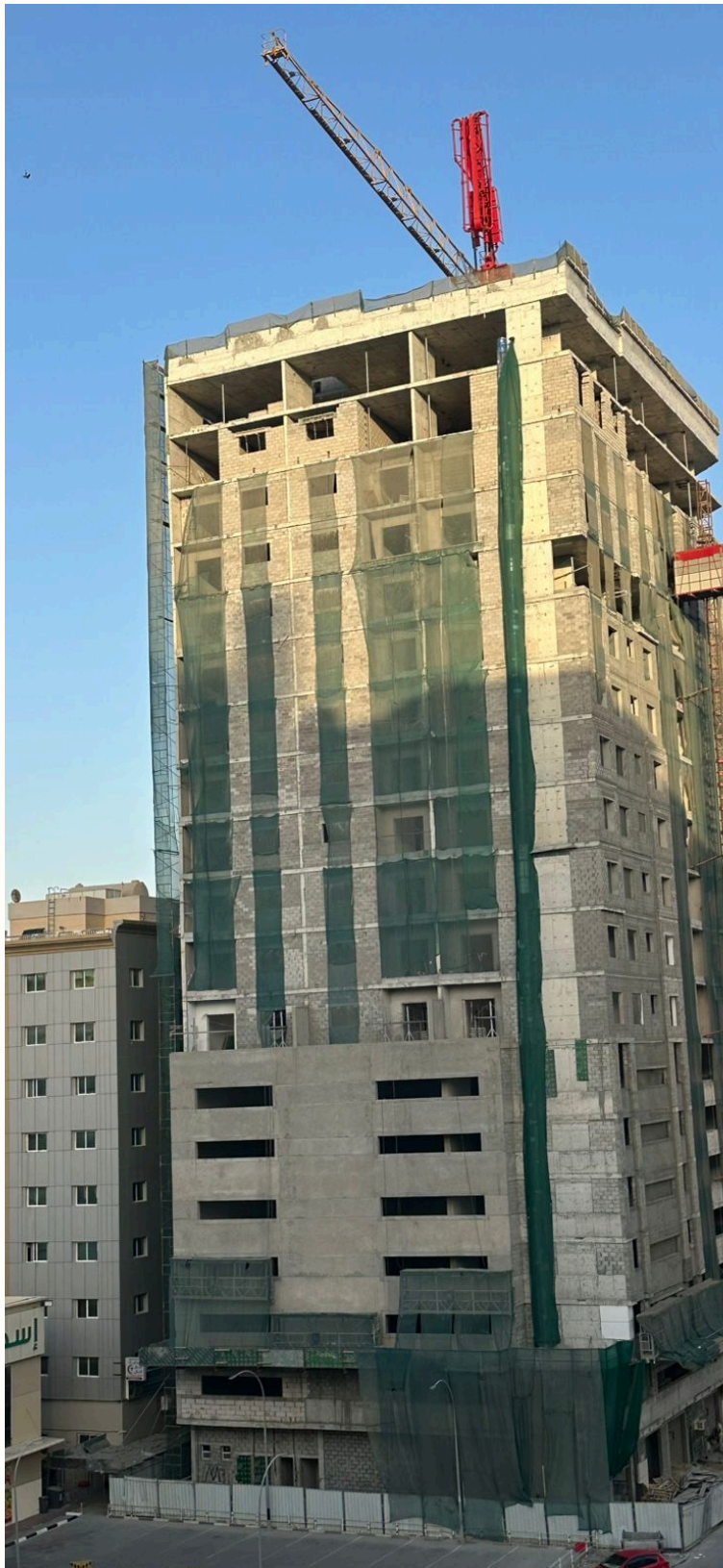
— High-rise structure — frame under construction
