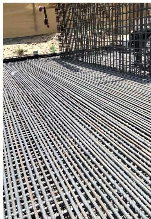
— Raft foundation reinforcement — bottom and top mats
