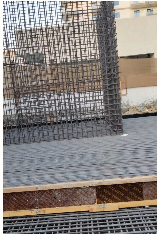
— Column starter bars — raft foundation
