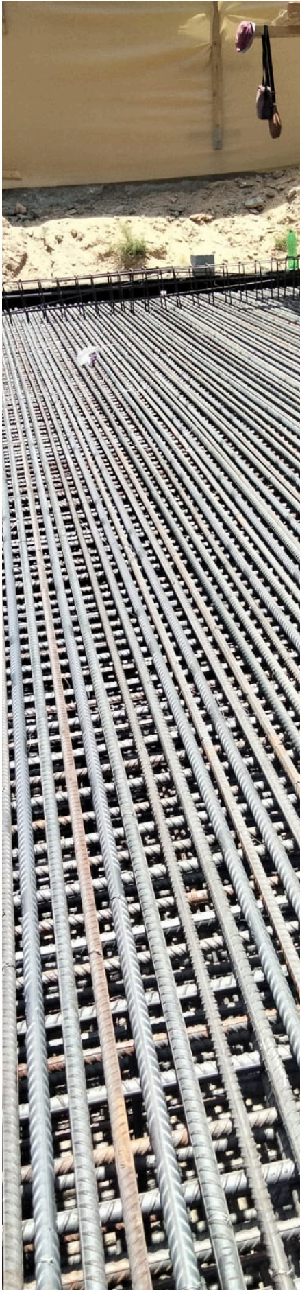
— Raft reinforcement mat, fixed and ready for inspection
